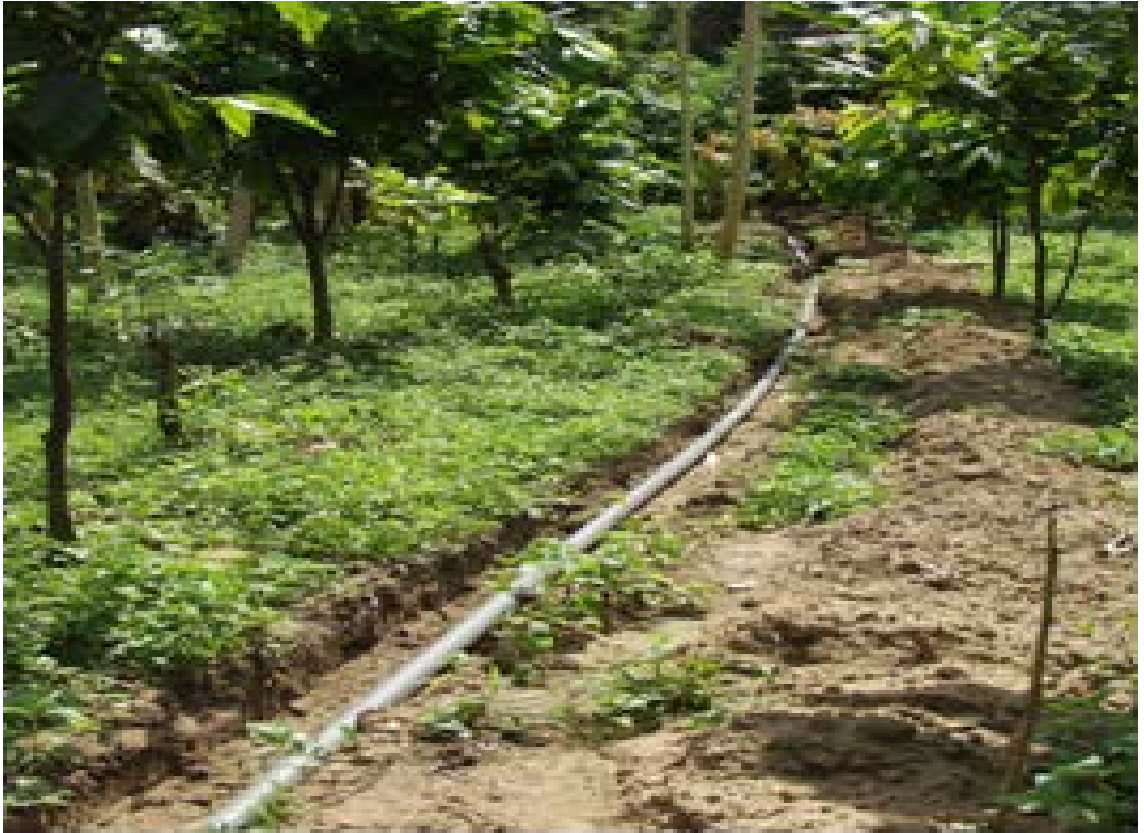
Plate 16 Inlet pipe from the dam
