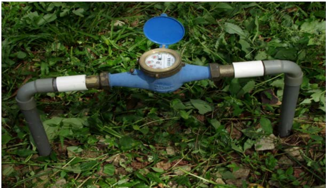
Plate 20 Meter for estimating quantity of water supplied through the outlet system
