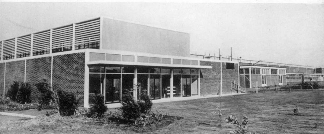
The new Rowntree factory, Melbourne, Australia.
